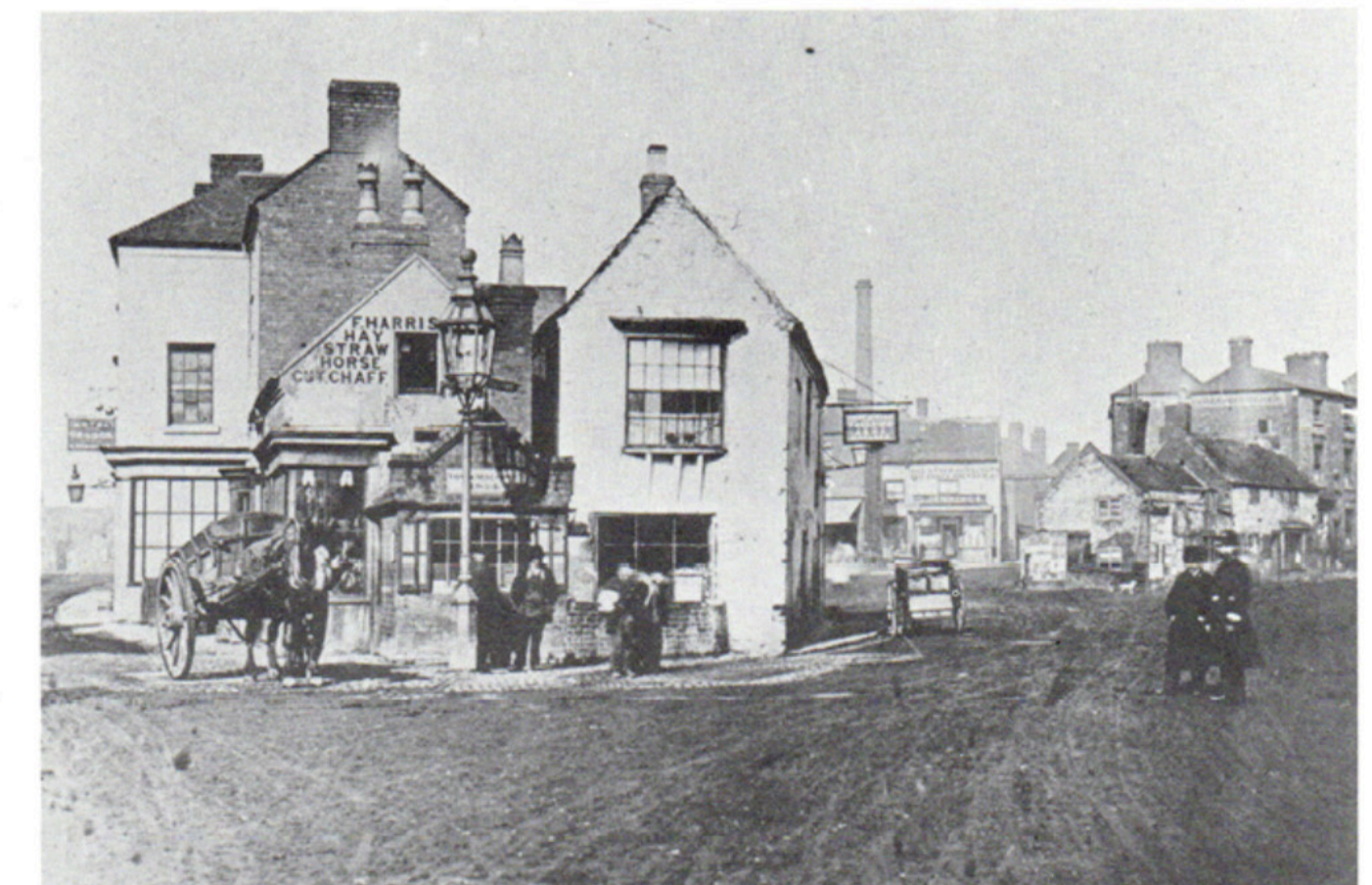
The horse still features in this 1875 photograph of Townend Bank, close to Park Street Wharf. Although the railways were now a faster, more popular way of travelling, the horse and cart was still used for hauling goods short distances. (Note also the inscription on the gable end for a dealer in hay, straw and cut chaff for horses.) But by now the whip makers and saddlers were starting to turn their attention to overseas business.
